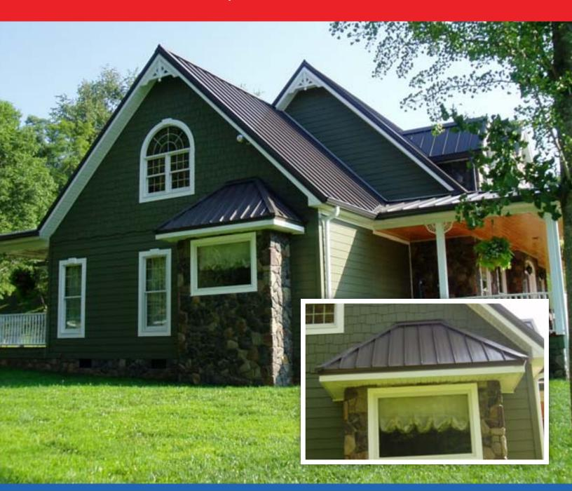
Custom fabricated "feature" metal roof panels by LifeTite exhibiting narrow o/c ribs for a more compatible aspect ratio
